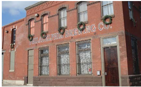
Example of a typical industrial building, now in use as a popular brewery, that will be seen on a walking tour that the East Kensington Neighbors Association is producing.
