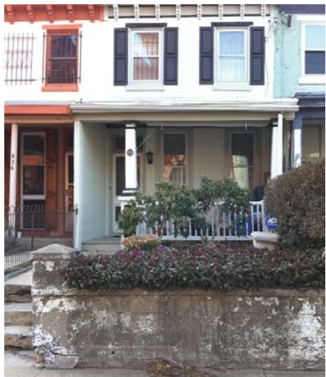
House in Fairmount before improvements.
