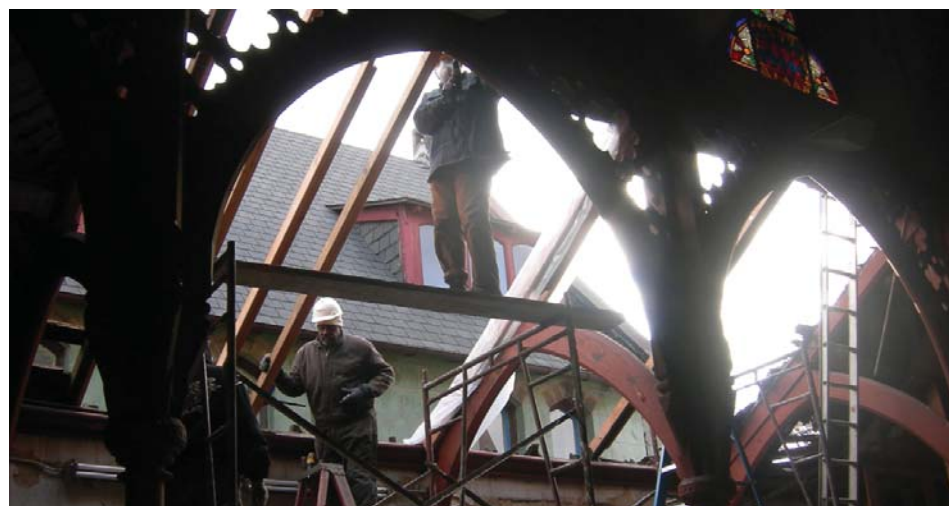
Emergency roof repairs being made by volunteers.
