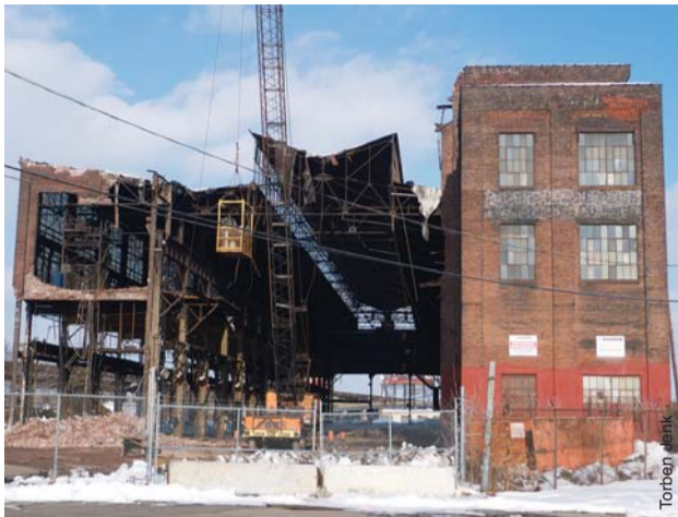
Cramp Shipyard Machine Shop No. 2
