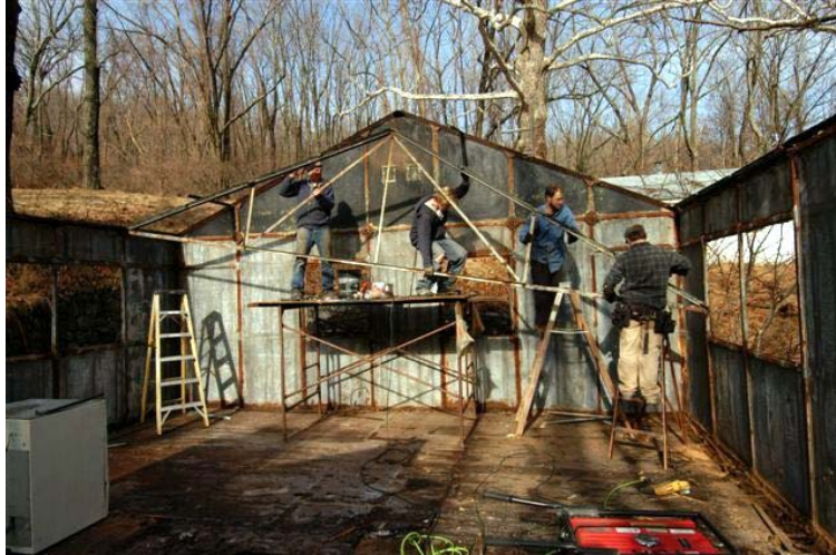
Disassembling the steel house. Photo: Dale Frens
