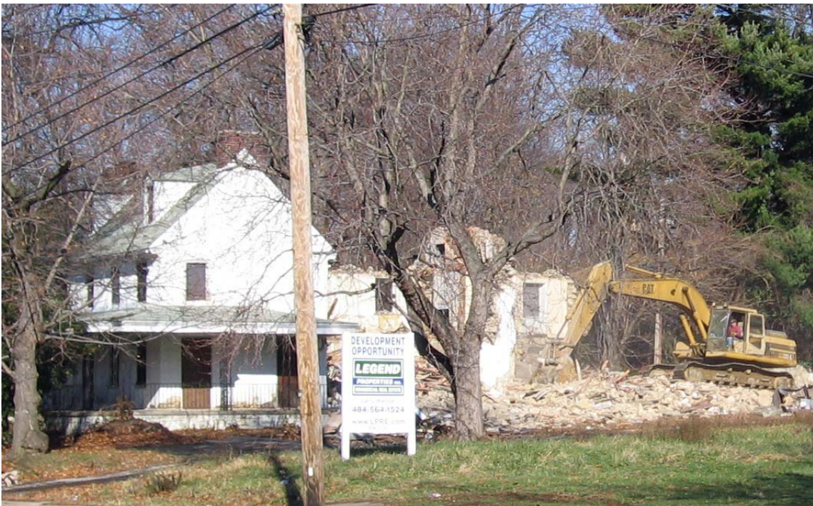
Bunting house being demolished
